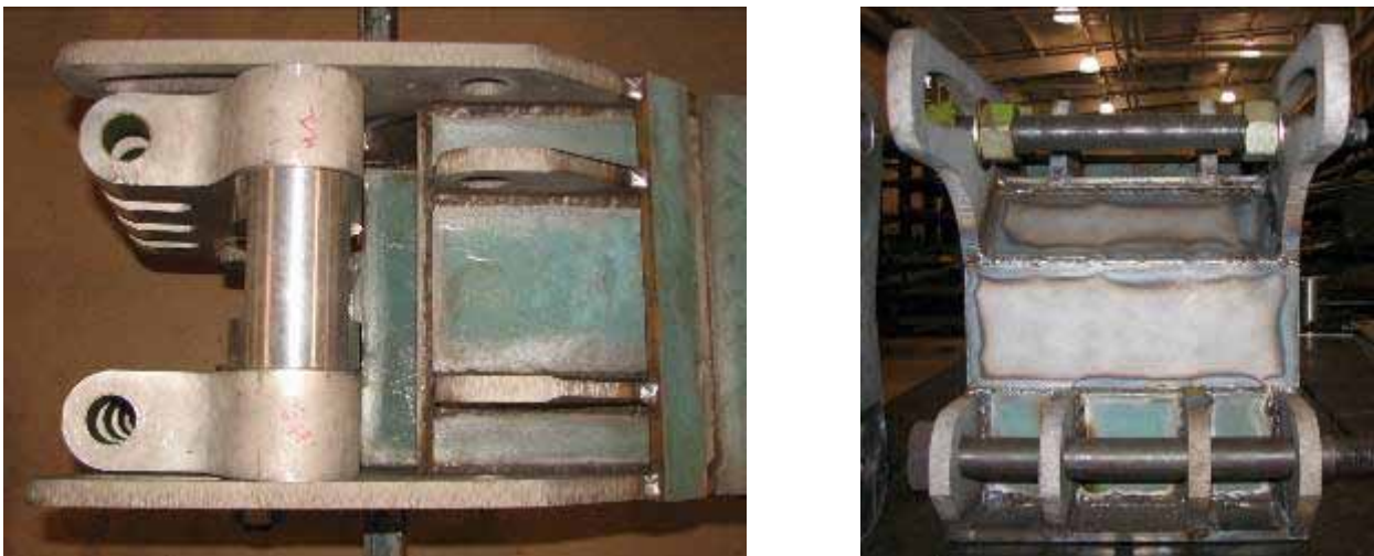
Figure 4.20: Left: 8 th and 9 th steps have been completed and jiggling has been removed. Right: 12 th step has been completed; cover plates were welded in place. Note: Jigs holding the Lower Adjustment Brackets should be left in when welding is taking place on the Inboard Beam. Free play tolerances were lost when those jigs were removed and welding operations performed.
