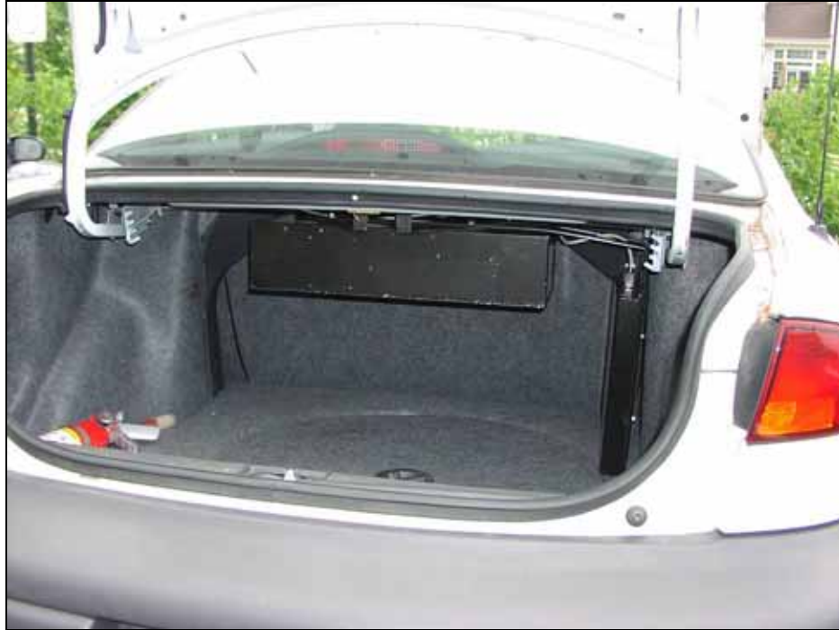
Figure 1.2. The main DAS unit mounted under the “package shelf” of the trunk.
