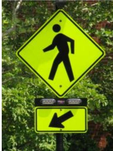
**Figure 23. Rectangular Rapid Flashing Beacon. (Source: Carol Kachadorian).**
