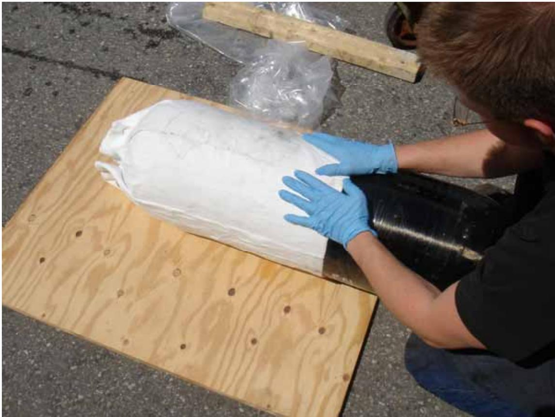
Figure 16 – Application of wet felt wrap to tank
