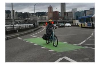
Figure 12. Dashed lines and green paint are used at this complex intersection in Portland, Oregon. (Source: pedbikeimages.org / Shawn Turner).
