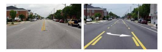
Figure 24. "Before" and "After" picture from a typical four-lane to three-lane conversion. (Source: Federal Highway Administration).
