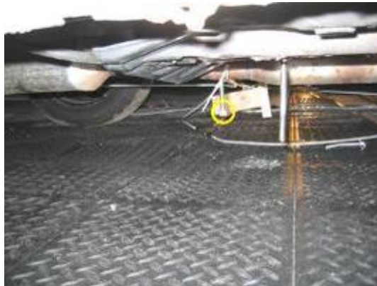
Figure I-10. Hydrogen leak straight down from tank position underneath automobile.
