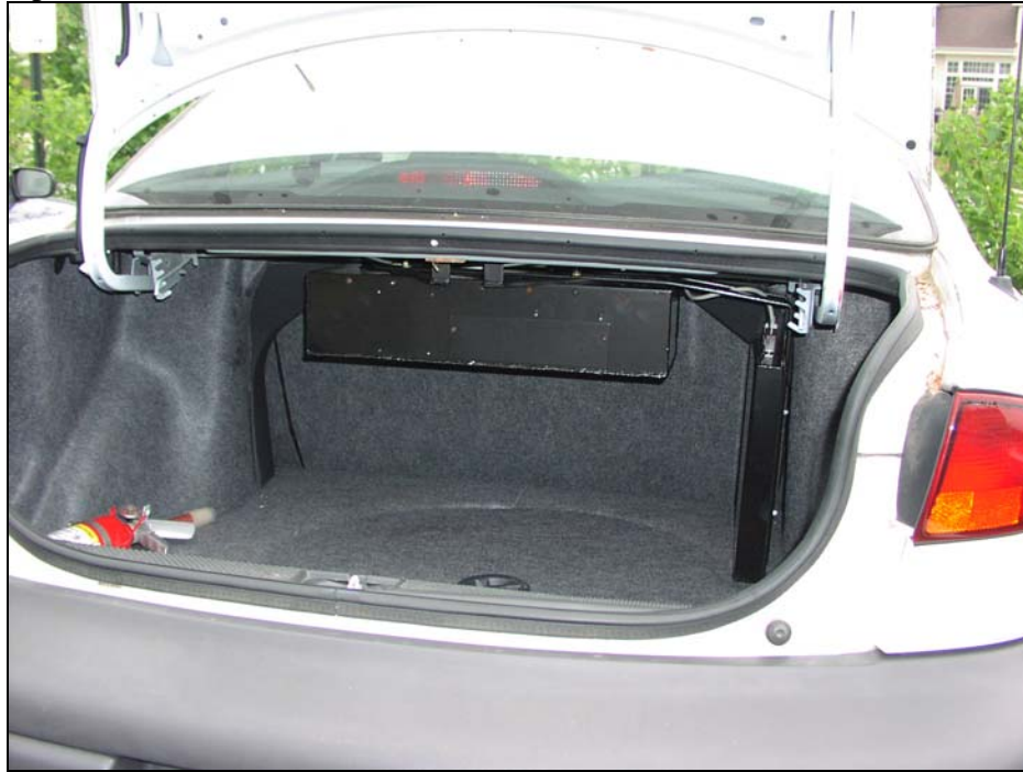
Figure 11. The Main DAS Unit Mounted Under the “Package Shelf” of the Trunk
