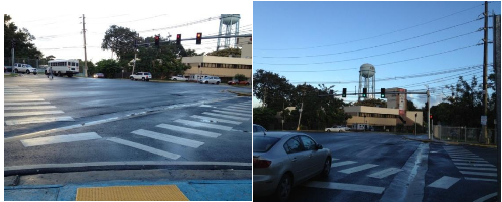
New Pavement Marking (Crosswalk) and Accessible ramps for pedestrians and people with disabilities
